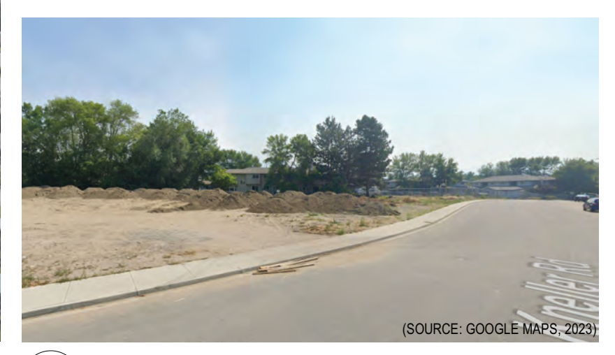
2 VIEW 2: VIEW OF NW CORNER OF SITE FROM KNELLER ROAD (DP-A1.01) N.T.S.
